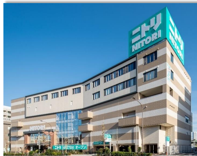
Nitori Meguro Store New Construction
