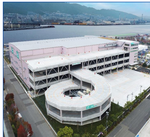
Nitori Kobe Distribution Center
