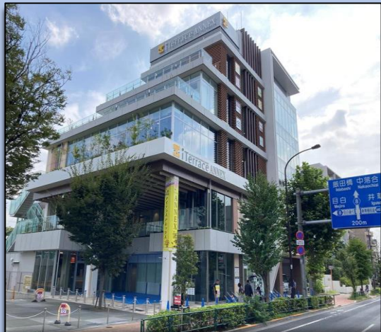
i-Terrace Ochiai-minami-nagasaki ANNEX
