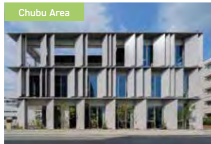
Chubu Area Crown Package Co., Ltd. Nagoya Sales Office [Aichi]
