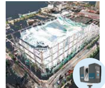
BIM modeling using a 3D scanner
